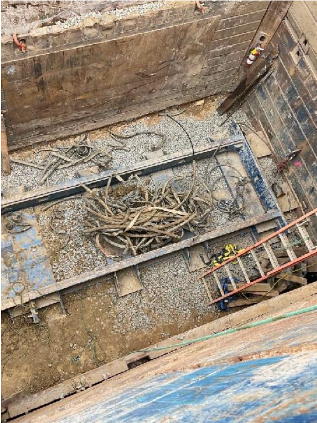
CenturyLink fiber line after being removed from auger.
