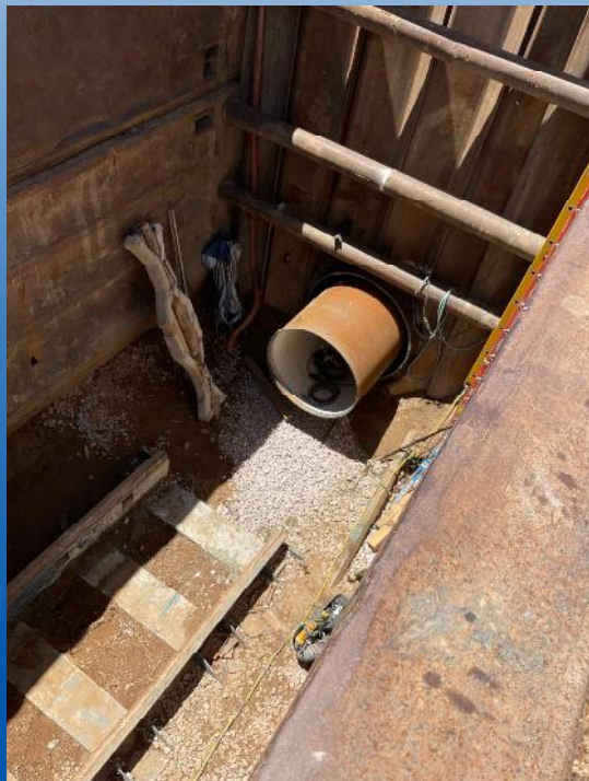
Installed 42" Carrier Pipe STA 71+00 – BNSF RR July 2, 2024
