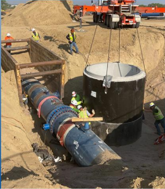
BFV and Vault Installation STA 289+79 – W of CR 5 July 31, 2024
