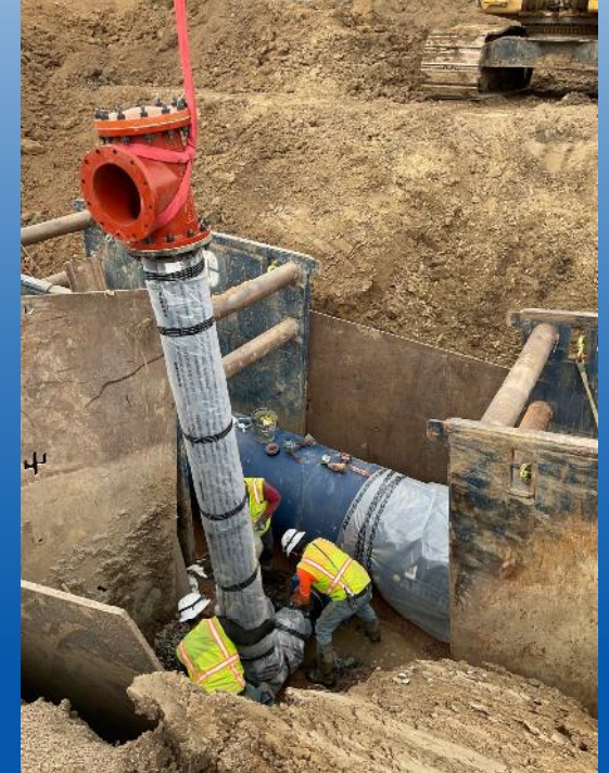
Blow-Off Installation STA 189+95 – W of CR 5 June 26, 2024
