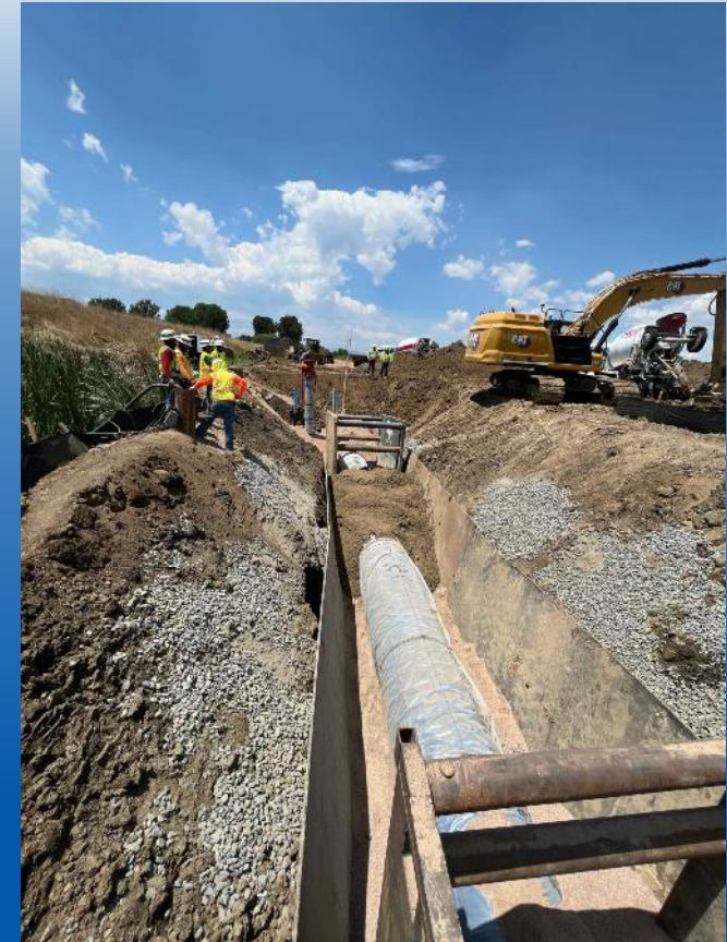
No-Name Ditch Crossing STA 266+70 June 26, 2024
