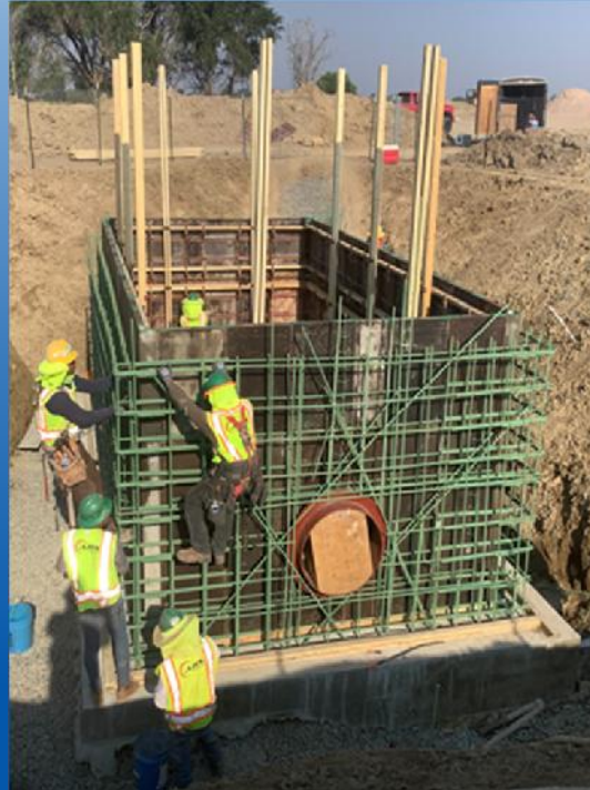
NWCWD Meter Vault Construction STA 296+00 – W of NCR 1 July 11, 2024
